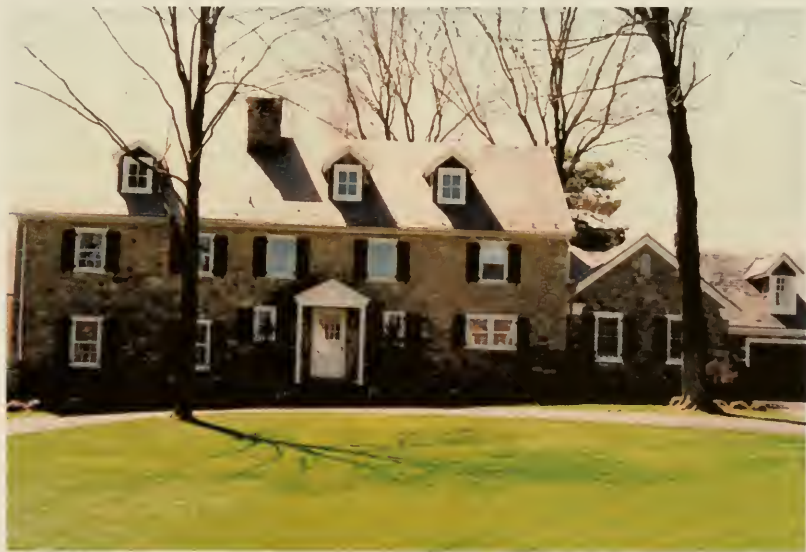
Photograph #26: The William Cox House (c. 1802) in Willistown Township. The serpentine for this house came from a quarry originally part of the same farm property.
